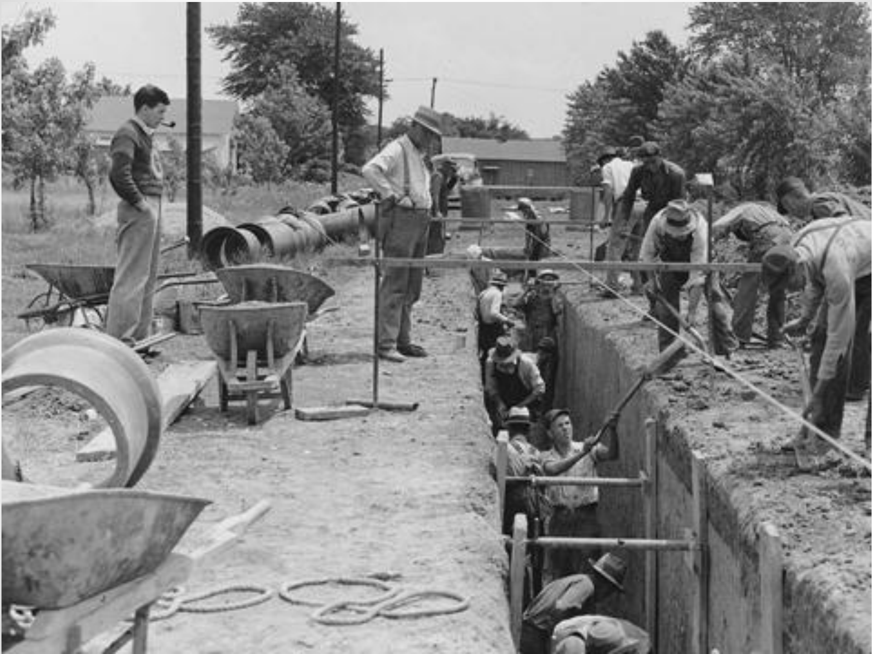
Men working on combined sewer line during Works Progress Administration 1934-1942
